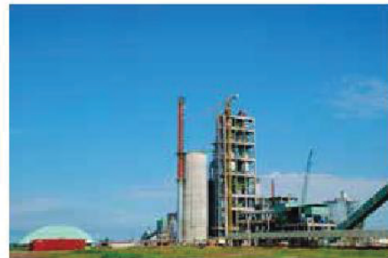
Binh Phuoc Cement Plant
