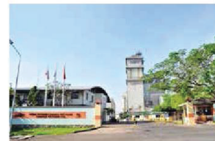
Cargill Binh Dinh Factory
